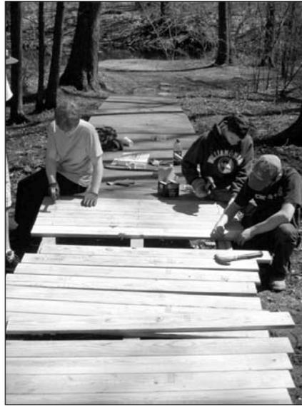
(Left) Area view including repaired plank footbridge (Right) Assembling the decking
