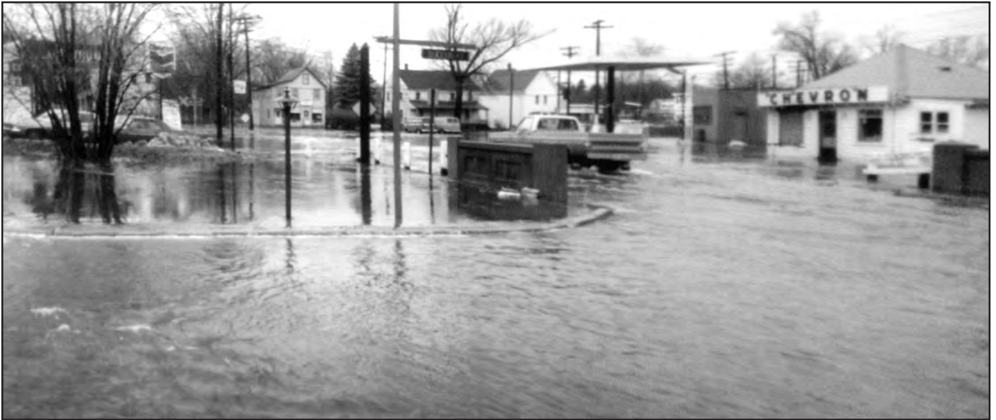
Looking west from the south side of School Street and Queens Way (where the Walgreens' plaza stands today). The image was submitted by Sue Lewis as three separate 3 x 3" photographs. Lynne Damianos combined them into this panoramic view. © Sue Lewis.
